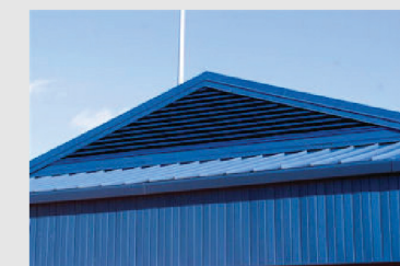
Roof/Ceiling-Space Vents.
